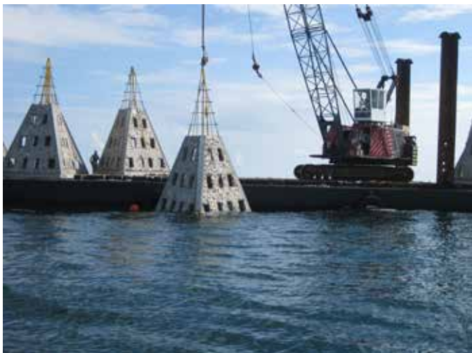
Concrete tetrahedron reef modules deployment.
